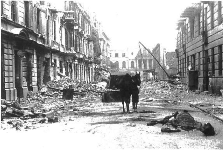
Collapsed streets of Warsaw, March 6, 1940.
