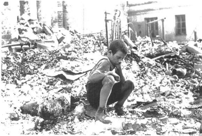
The young Pole has returned to where his house once was, now turned into ruins during a break in the shelling from the air in Warsaw in September 39th.
