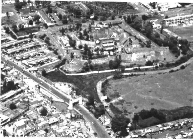
Road connecting Peshawar-Torkham
